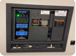
Replace your existing STR Trip Unit with confidence using the fully programmable, retrofittable, DM-1000 Electronic Trip Unit.
